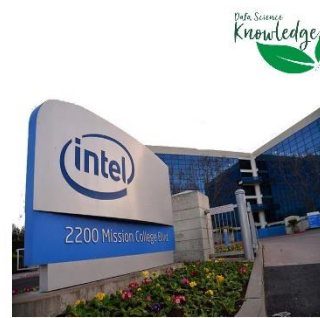
Intel headquarters, at 2200 Mission College Boulevard in Santa Clara, California. The objects on the roof are wind turbines installed in May 2015 as part of a green energy project.
